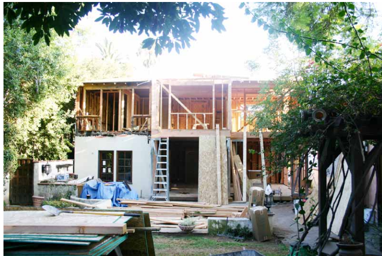
All the framing nearly done in less than a week...wow!
