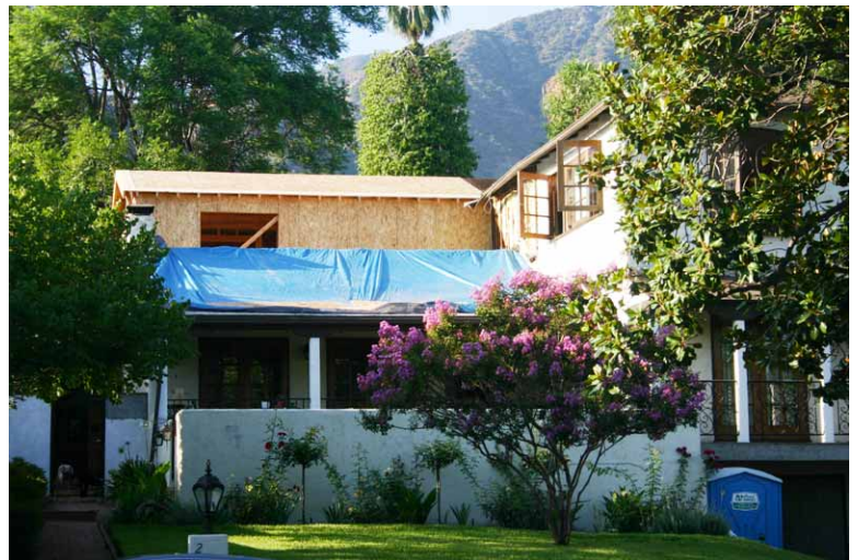
Street view of second floor addition.
